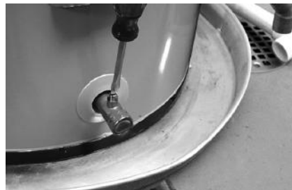
Figure 20 - Draining the old water heater.
