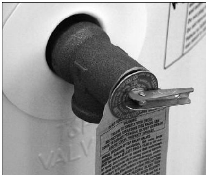
Figure 25 - Temperature and Pressure Relief Valve
