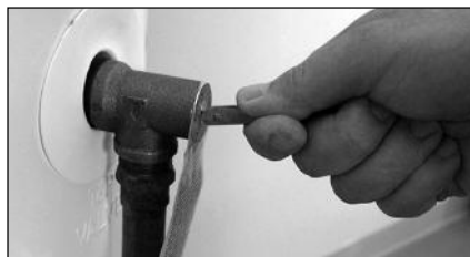
Figure 45 - T&P Relief Valve.
