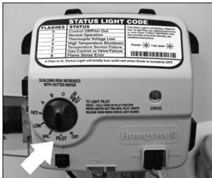
Figure 48 - Gas control/valve.
