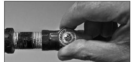
Figure 58 - Gas valve in “on” position.
