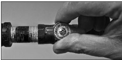
Figure 32 - Gas valve in "on" position
