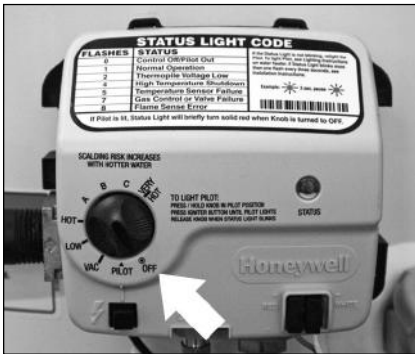
Figure 40 - Turn gas control/temperature knob OFF.
