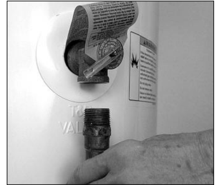
Figure 21 - Removing the T&P Relief Valve discharge pipe.
