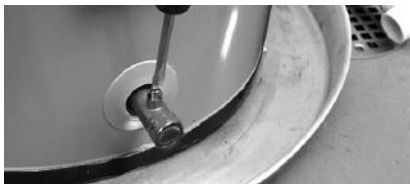
Figure 42 - Draining the water heater.
